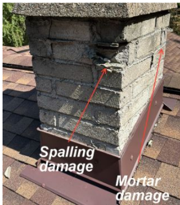
Brick spalling
